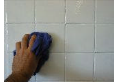
Clean and degrease the tiles
