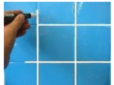
Renew the grout lines with Flag Grout Marker
